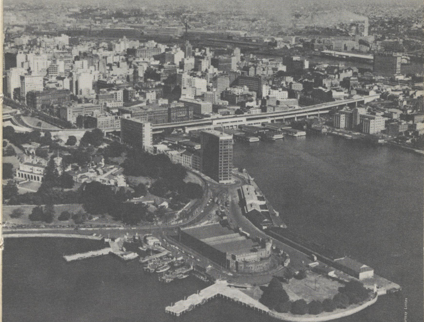
BENNELONG POINT LOOKING TOWARDS THE SOUTH-WEST
